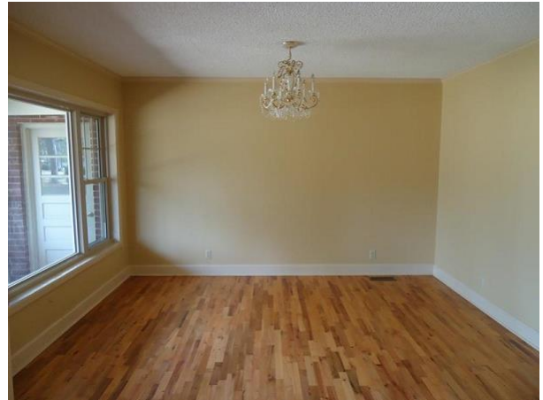
Typical photo with 3 walls
